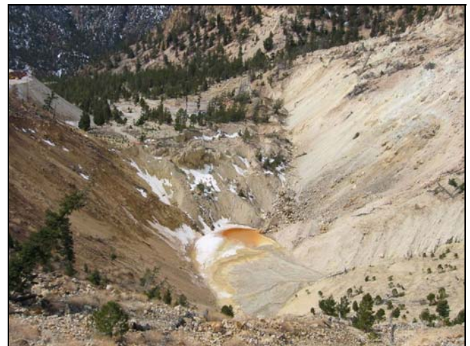
Figure 3. Center of Goathill Glory Hole in 2004 (view to southwest)
