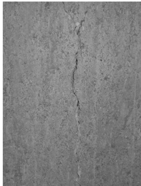
Figure 3c. Shaft #1—Vertical Crack Branching from the Main Horizontal Crack at 227 ft Below the Collar
