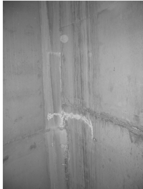
Figure 3b. Shaft #1—Horizontal Crack with Zero Offset at Patrician Wall 227 ft Below the Collar
