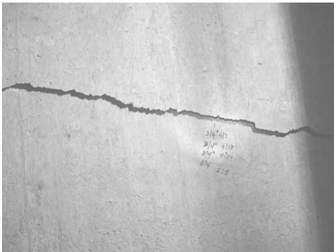
Figure 3a. Shaft #1—Maximum Offset from Shear Failure at 227 ft Below the Collar
