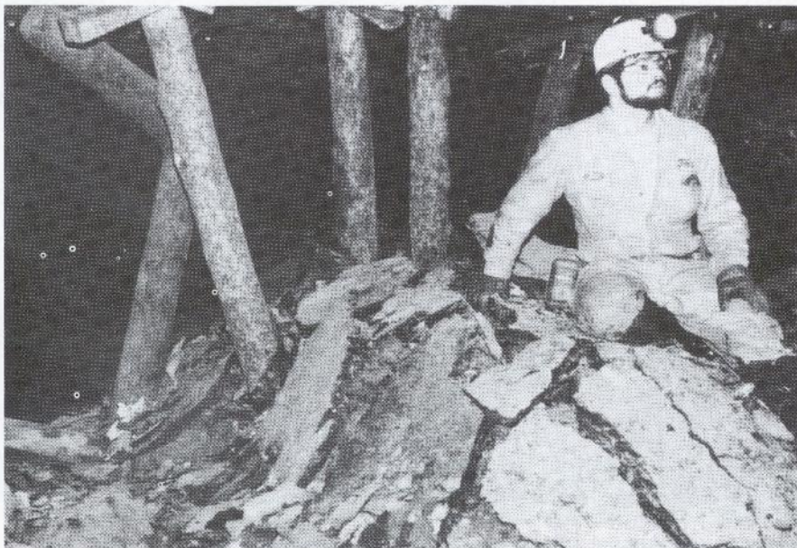
Fig. 7 — Typical floor heave behind the longwall face — Eighth left, room two.
