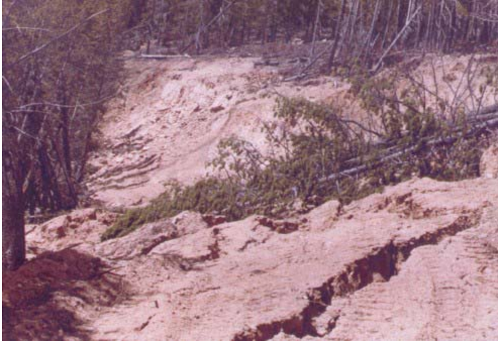
Figure 6. East wall headscarp following the March 1983 northeast corner slope failure.
