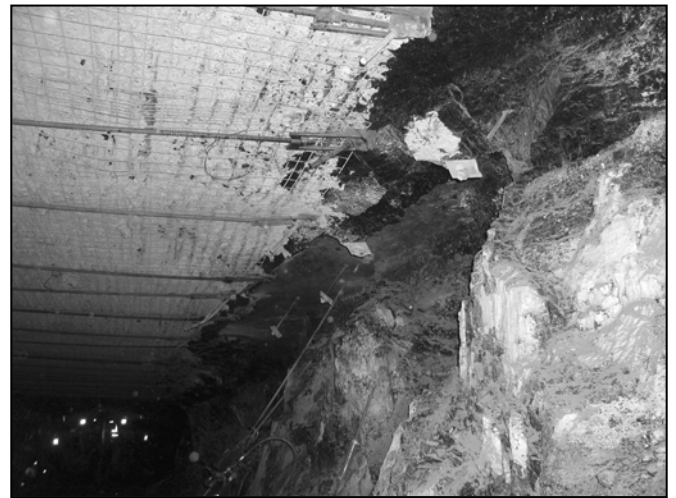
Figure 9. Horizontal Stress Damage along Corner of Roof
