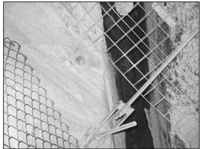
Figure 10. Open (15 cm) Aperture Along Fault Blade in Roof In Low Horizontal Stress Zone
