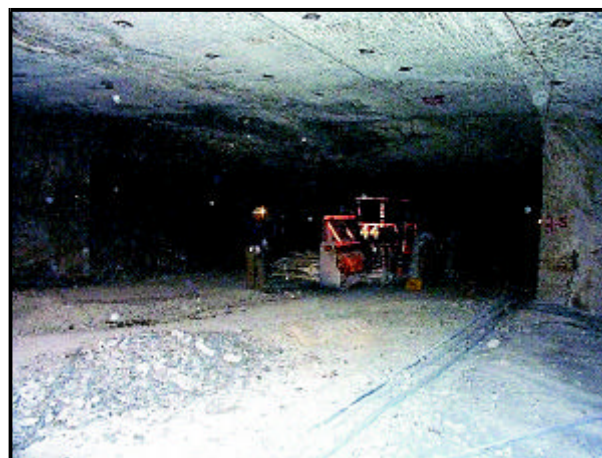
Figure 8. Typical Intersection in a Belt Entry
