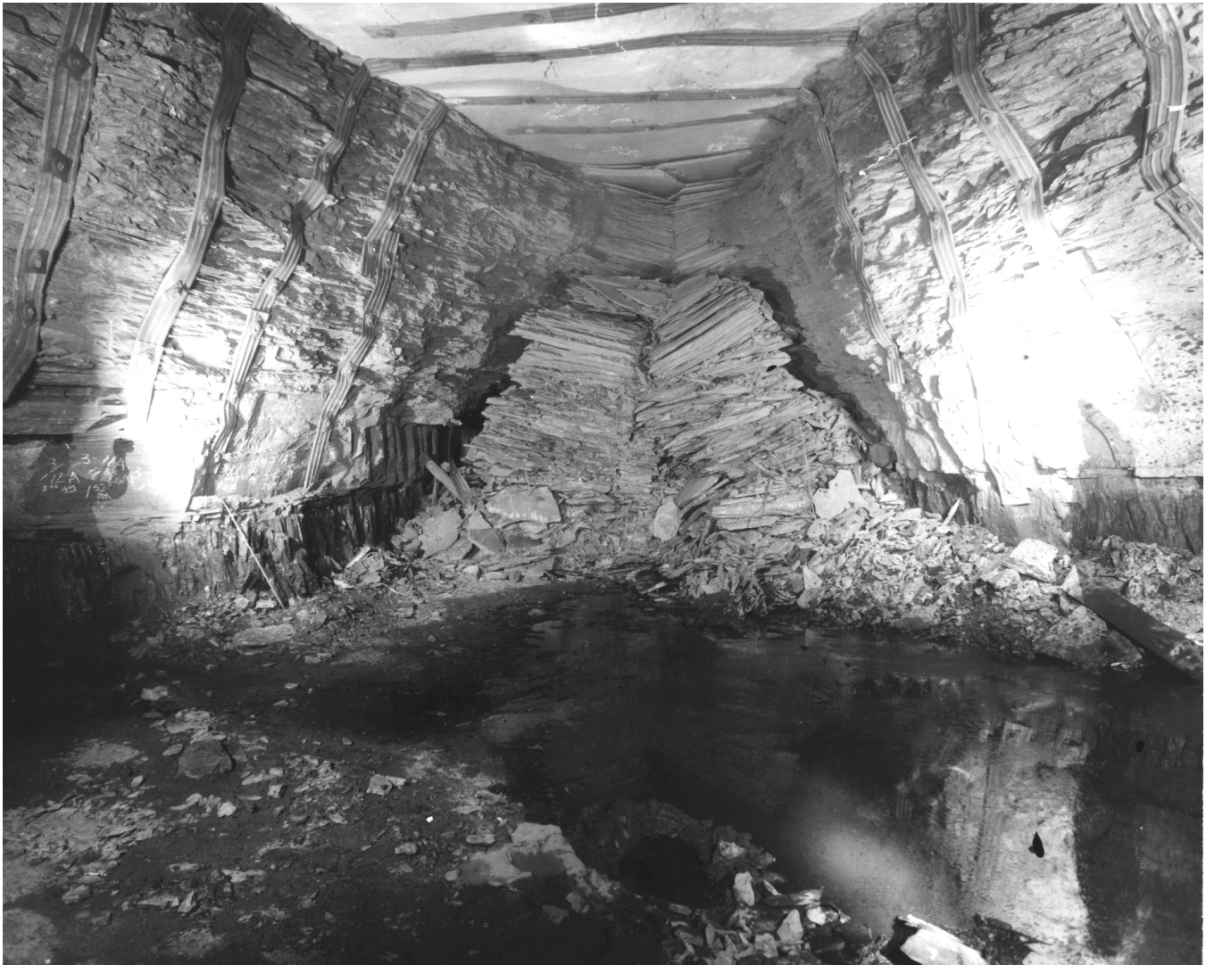
Figure 2. Beckley Mine Roof Fall
