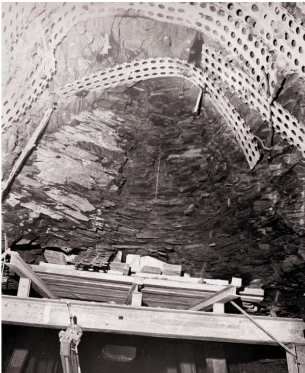
Figure 1. Dome of White Pine Roof Fall
