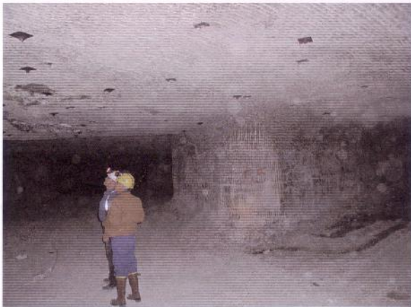
Figure 2. Typical Good Roof, Floor, and Pillar Conditions in a Beltway-Room Intersection
