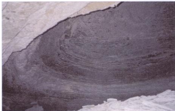
Figure 12. Roof Fall Induced by Gas Pressure
