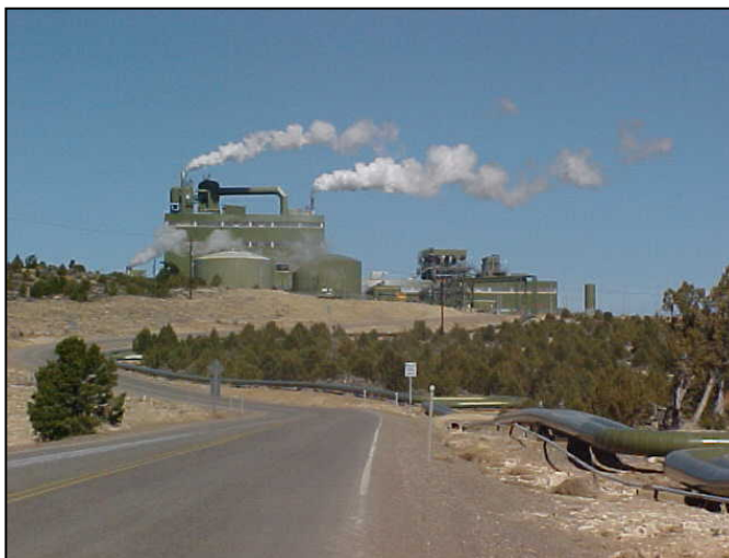
Figure 4. Upper Processing Facility
