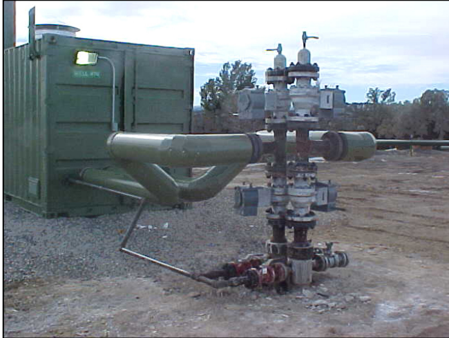
Figure 7. American Soda Wellhead and Instrumentation Skid
