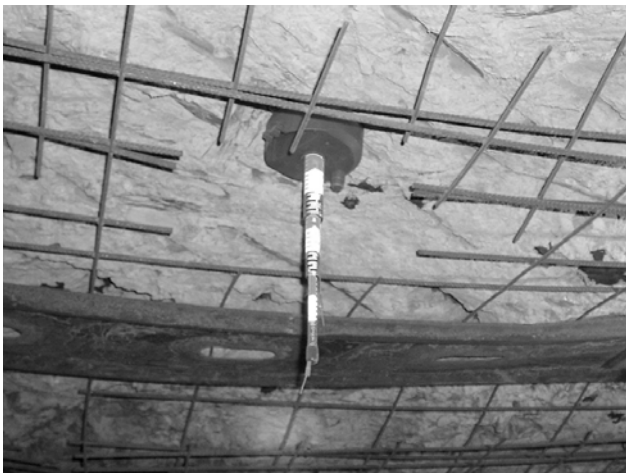
Figure 3. Three-Position Telltale Installation.
