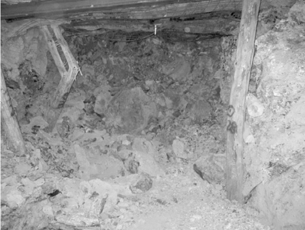
Figure 4. Timber Posts Broken By Pillar Convergence.
