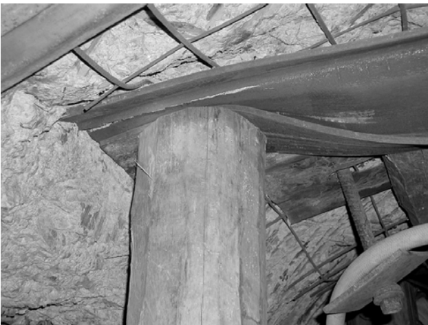
Figure 5. Crushed Steel Beam Resting on Timber Support.
