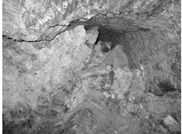
Figure 6. Plastic Deformation of Manto into the Mine Opening.
