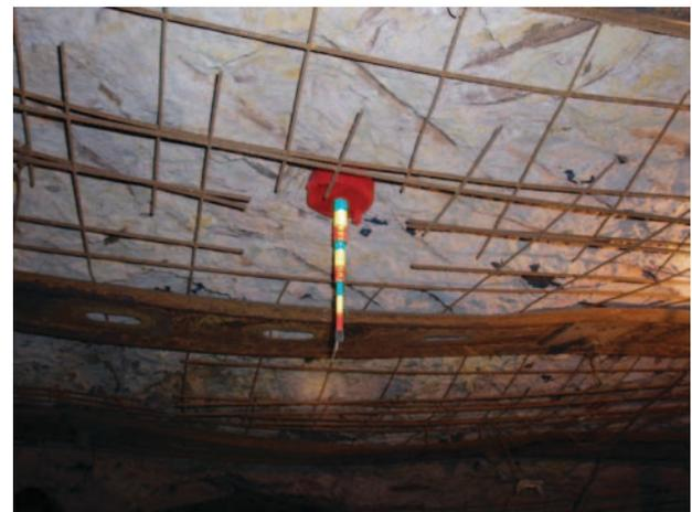
Figure 4. Typical installation of triple height telltale.
