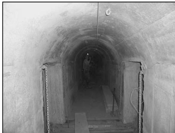
Figure 12: Typical Draw Line after Liner Construction
