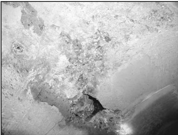
Figure 15: Void in the Concrete Liner near the Crown Caused by an Incomplete Pour
