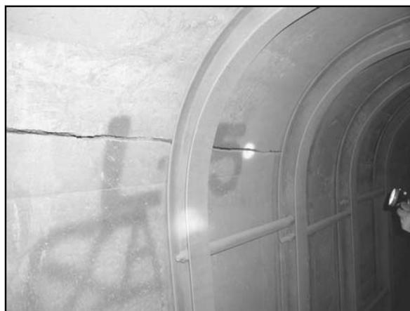
Figure 13: Horizontal Tensile Fracture at a Concrete Cold Joint and Precautionary Steel Sets in a Draw Line
