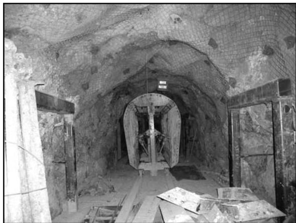
Figure 11: Draw Line Development Showing Original Excavation and Concrete Forms
