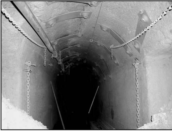
Figure 14: Compression Cracking and Straps along the Crown of a Draw Line
