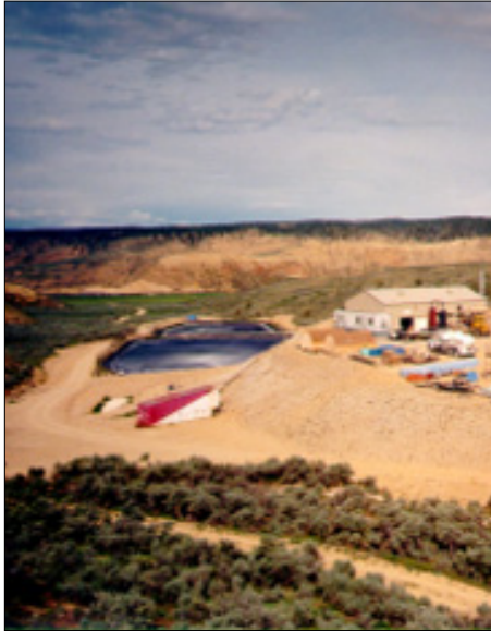
Figure 4. Pilot Plant Area
